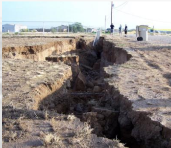
Earth fissure generated by water extraction in Mexico City
