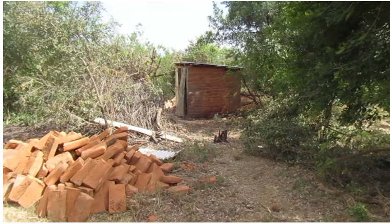
Shower and latrine module
