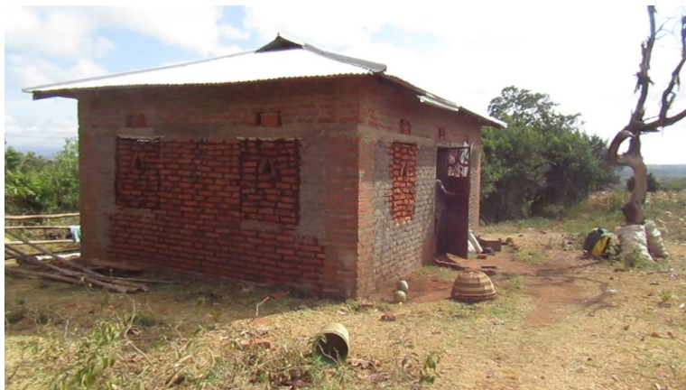
Nico's brick house: still under construction.
